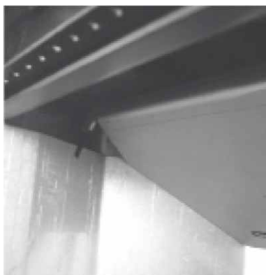
Figure 12. Lift the fire protection plate
