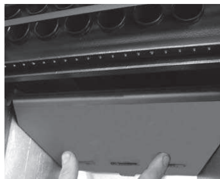
Pict. 14: Lift the fire shield
