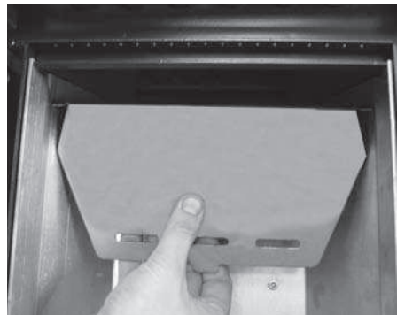
Pict. 16: Rotate the fire shield
