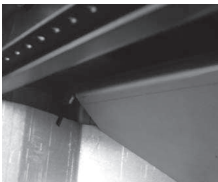
Pict. 15: Lift the fire shield
