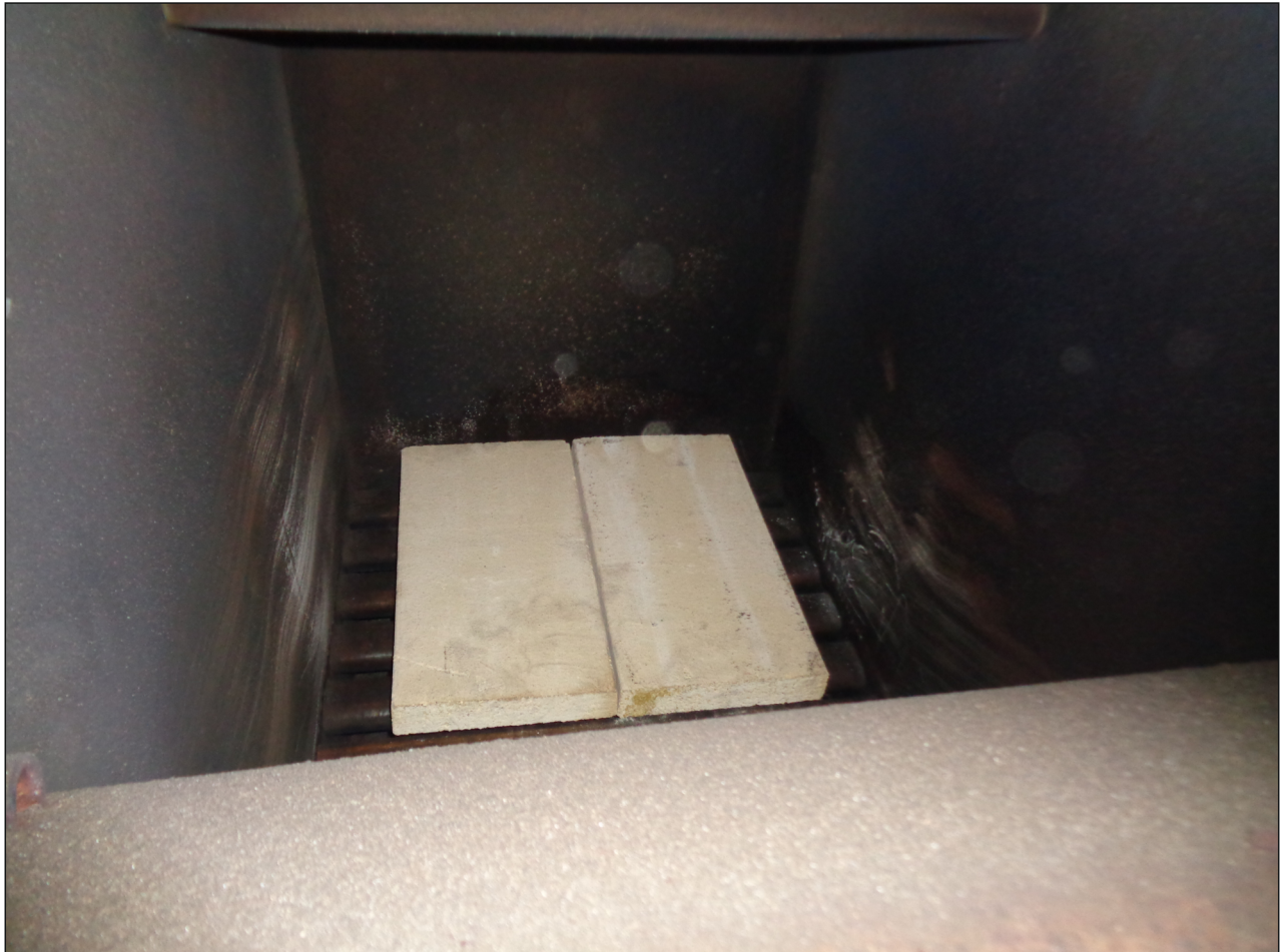
Picture 5: Position of fireclay plates on top of the grate in the firebox.
