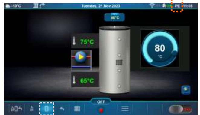
Accumulation (buffer) tank screen (PE)
