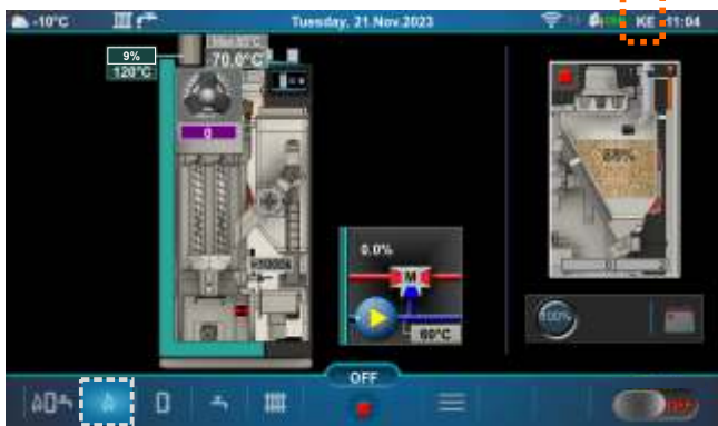
Boiler screen (KE)
