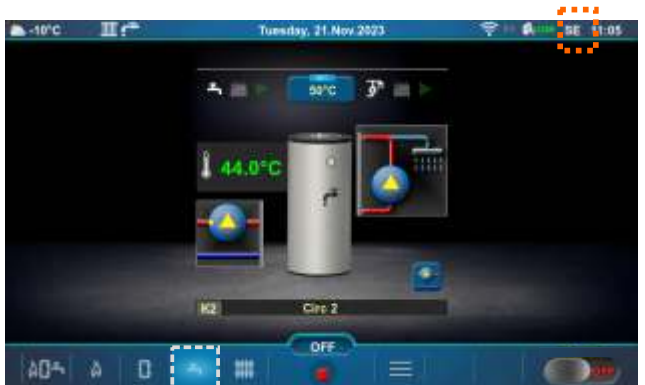
Domestic hot water (DHW) tank screen (SE)
