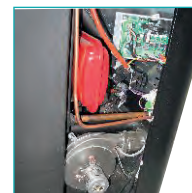
Expansion vessel, flue gas fan
