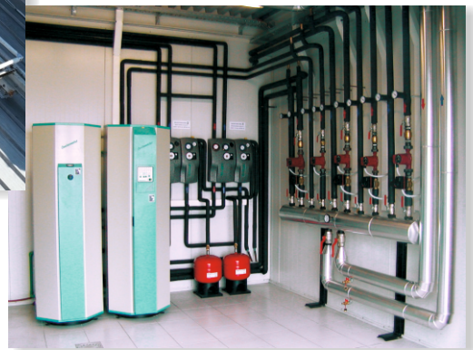
An example of a built-in educational/demonstration solar system with two separate collector circuits (flat CPK 8203N 4H and tube vacuum CVSKC-10), one solar boiler STEB and one storage boiler TB, solar pump groups and all necessary fittings.
