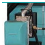
Pellet burner on the boiler
