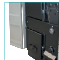
Boiler door, thermomanometer, draft regulator
