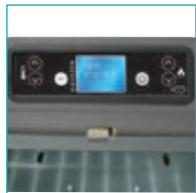
Boiler controller (can be installed on the left or right side of the boiler)
